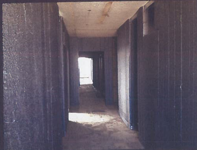
The interlocking, graphite-infused, expanded polystyrene (EPS) panels used in the project are a distinctive charcoal colour, unlike the snow white colour of standard EPS panels
